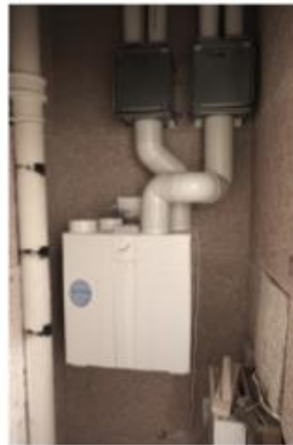
MVHR installed into an existing cupboard lined with wood wool, lowered ceilings in halls to conceal ducts
