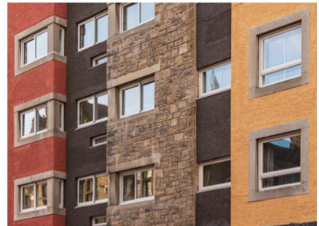
Repairs to render, repointing, and redecoration to match original colours
