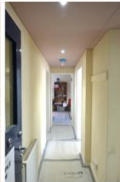
MVHR installed into an existing cupboard lined with wood wool, lowered ceilings in halls to conceal ducts
