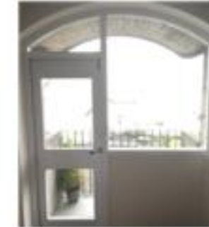
Replacement window and door screens installed
