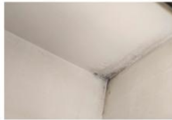
Mould occurring along a thermal bridge
