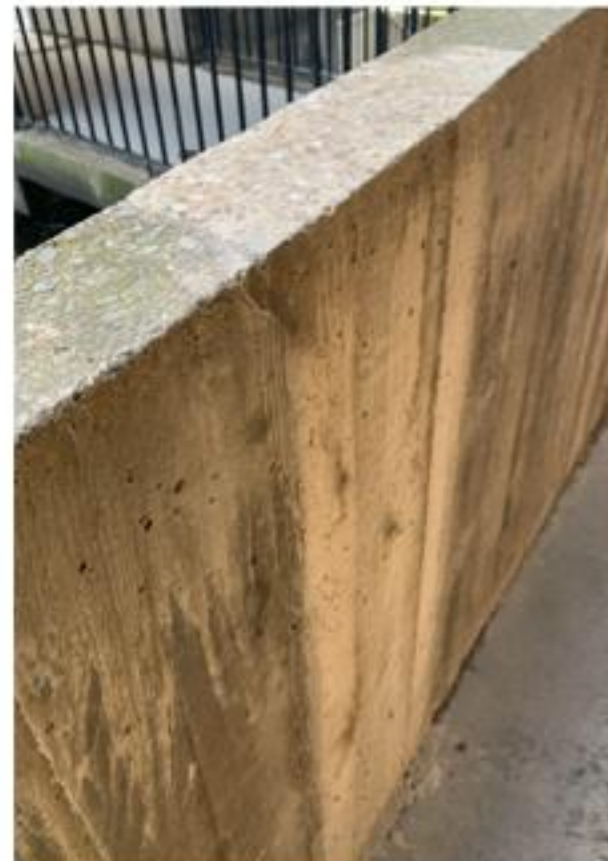
Repairs to cast in-situ concrete completed
