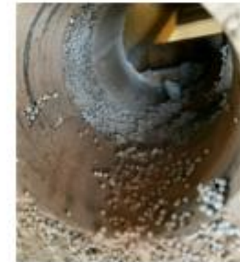
Cavity wall insulation
