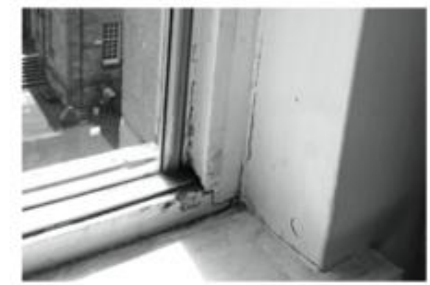
Single glazing condensate rotting frames
