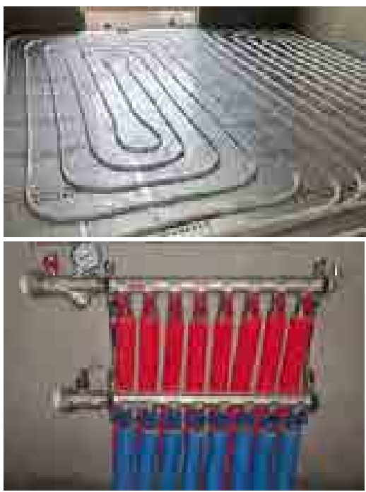
Under floor heating system installed on both floors
