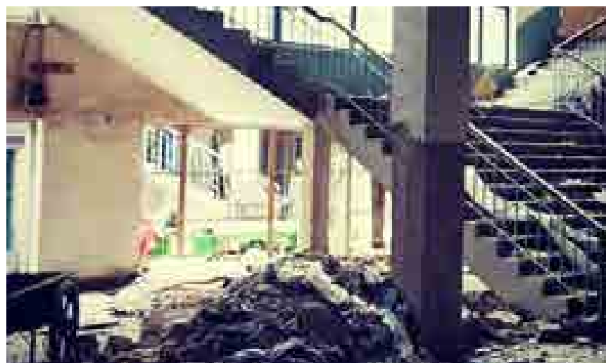
Exposing the concrete columns
