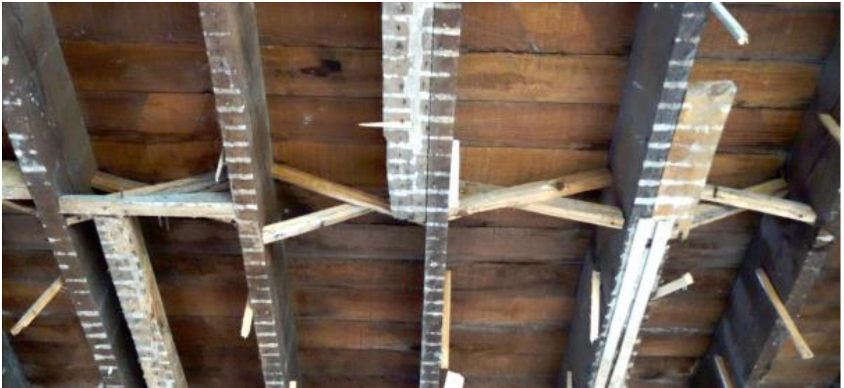
Figure 22 X-shaped timber connections between the timber joists
