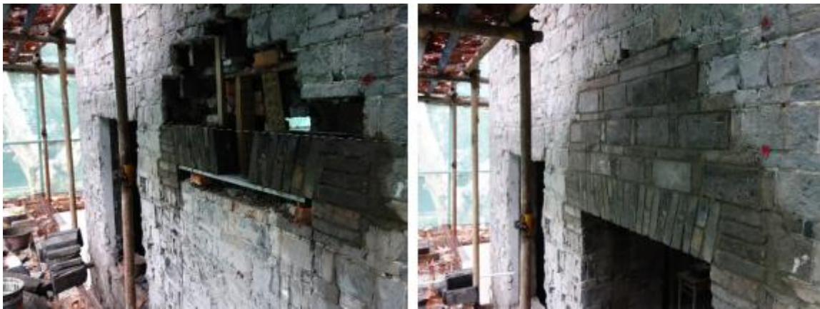
Figure 16 Before and after the repair of an opening
